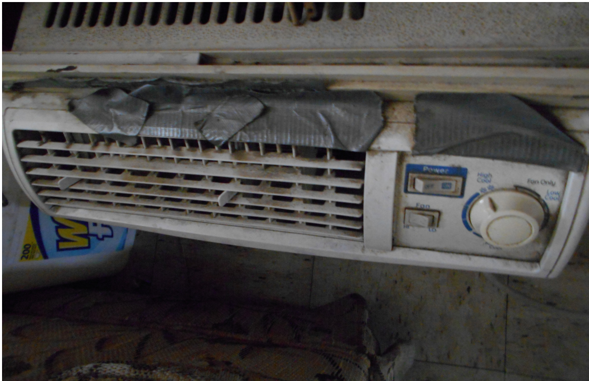
Photo 40 - A window air condition that is dirty and covered in tape
