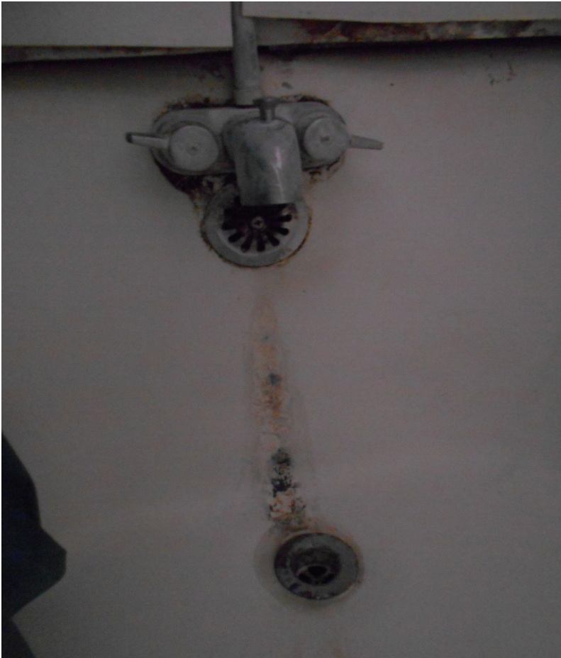
Photo 16 - A bath tub with unknown black/brown substance, dirty, and missing pieces of the bathtub
