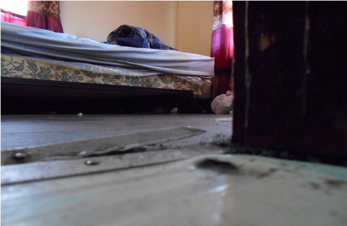
Photo 52 - Doorway into resident's room with broken metal jutting upwards
