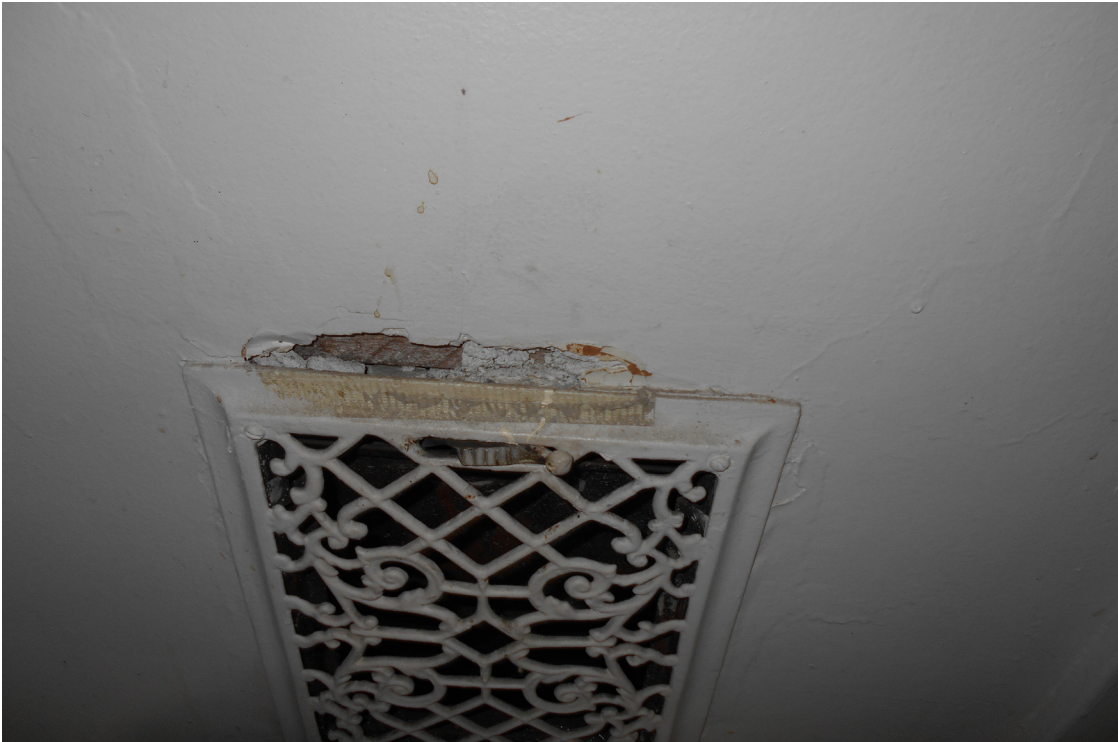
Photo 66 - Walls cracking/missing around vent
