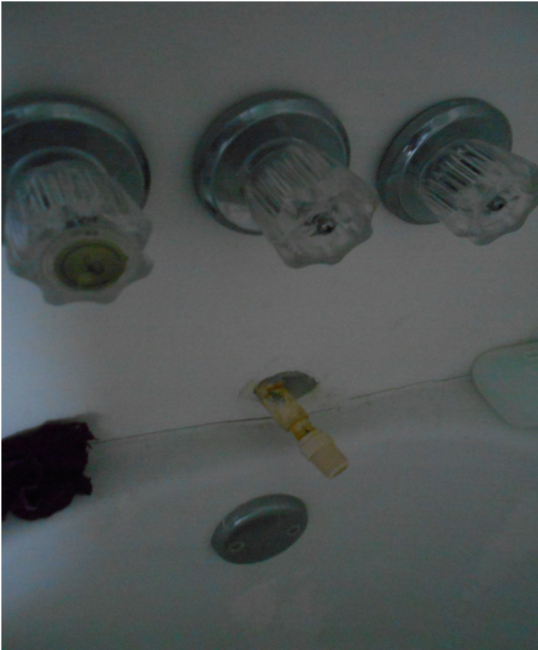
Photo 98- Bathtub with hose sticking out of it-hose appears to be the spout (no covering)
