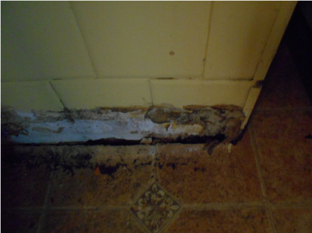
Photo 116- Kitchen molding missing-tiles broken and separated from floor-unknown black and brown substance present
