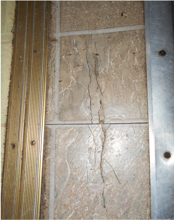
Photo 12 - Flooring in one of the houses-cracked/dirty
