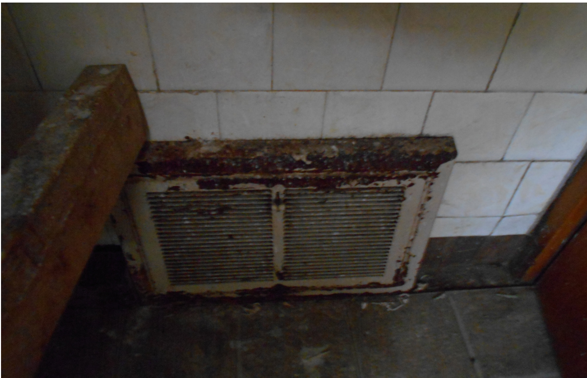
Photo 37 - Vent in bathroom that is covered in unknown substances and rusted
