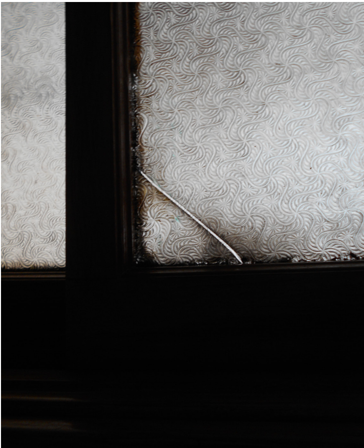
Photo 31 - Crack in a bathroom window
