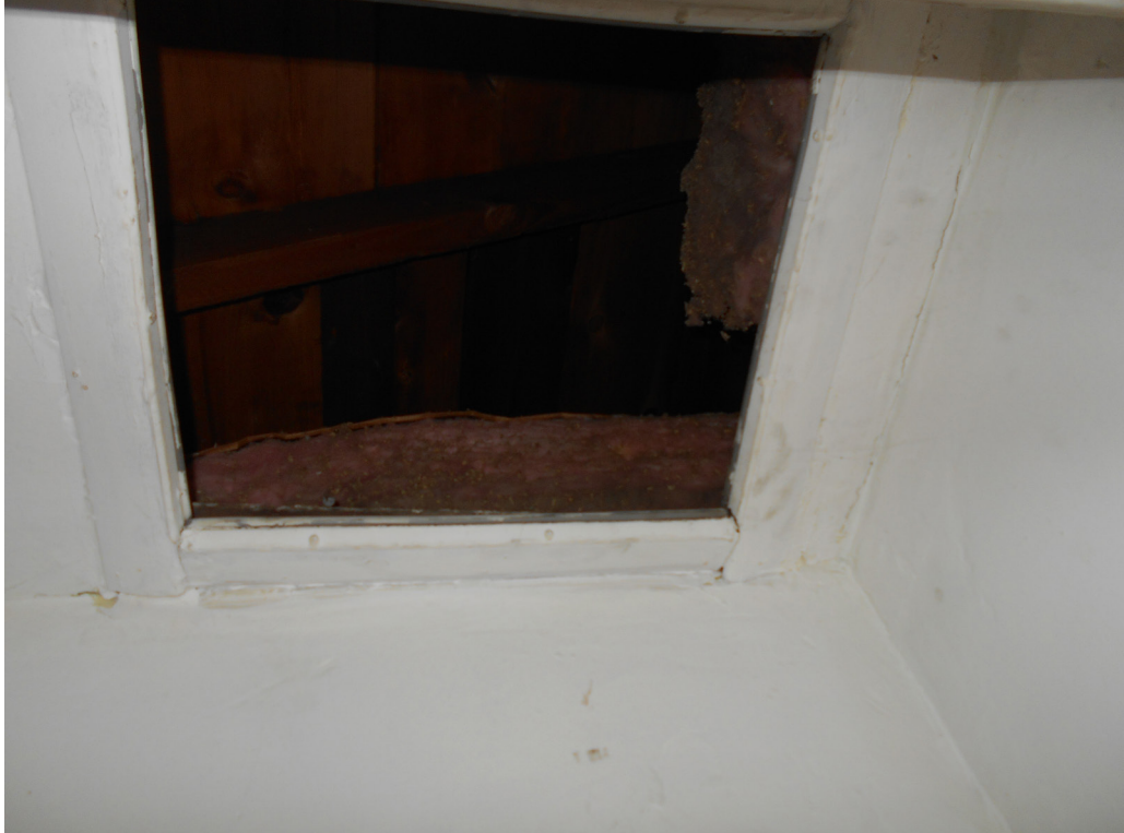
Photo 87 - Hole in resident's closet ceiling
