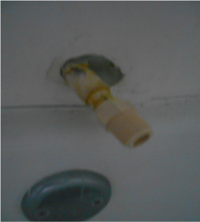
Photo 96- Exposed tube not covered by tub spout- missing piece of the bathtub
