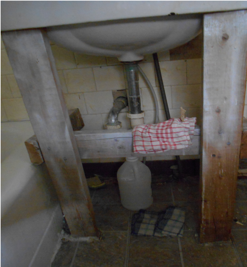
Photo 38 - Bathroom sink that is held up by pieces of wood/floor is dirty/missing tiles
