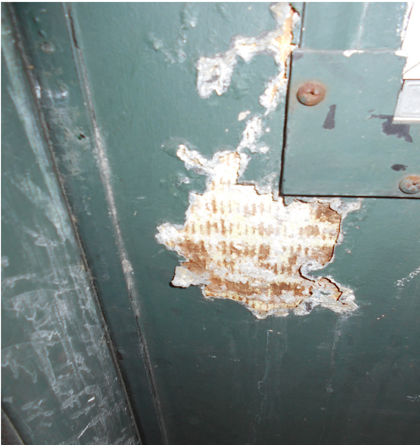
Photo 119- Door missing pieces of metal and rusting
