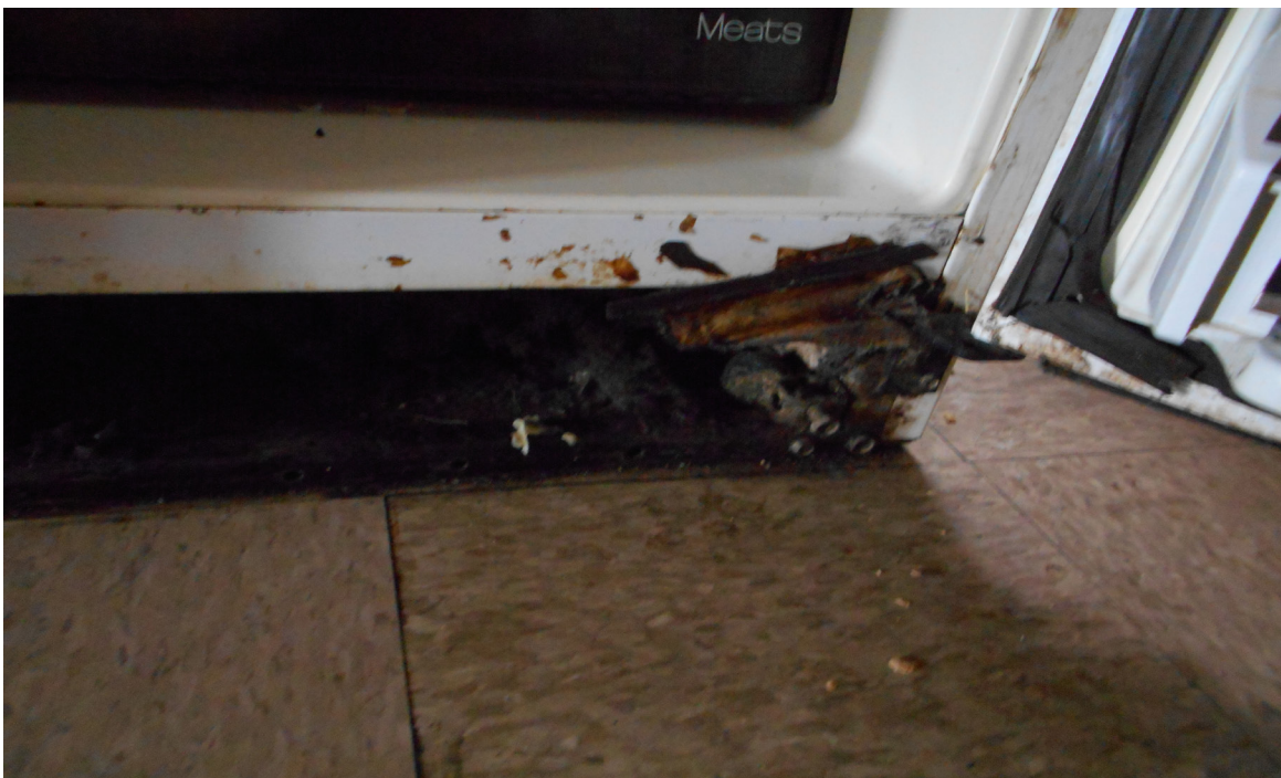
Photo 11 - Bottom view of the same refrigerator-dirty/rusted/holes
