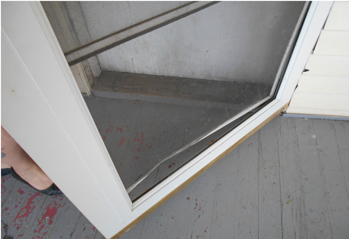
Photo 55 - Screen broken on front door
