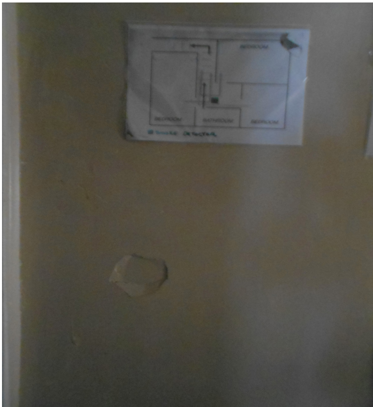
Photo-107- Hole in the wall of resident's room
