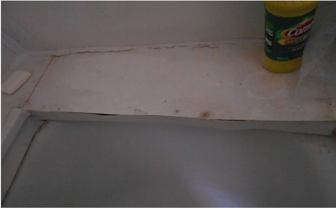
Photo 14 - Bathtub is missing molding/holes and there is evidence of an unknown black/brown substance
