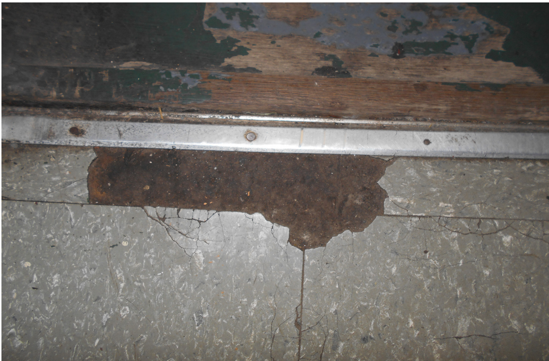
Photo 27 - Flooring in one of the homes that is broken/dirty/and missing pieces of tile
