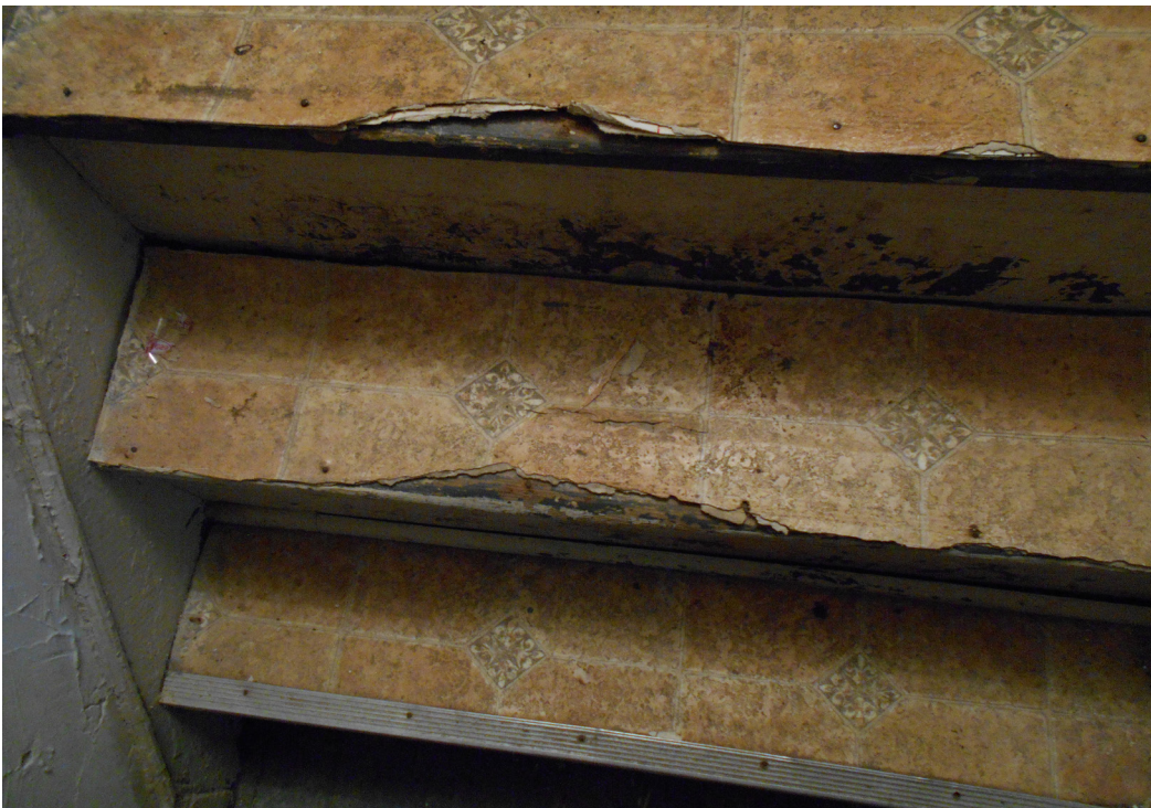
Photo 117- Flooring missing from stairs
