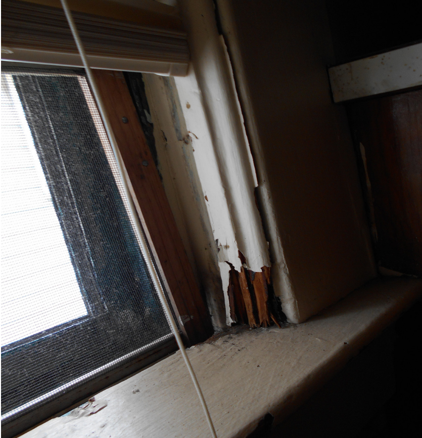
Photo 43 - A window frame - broken
