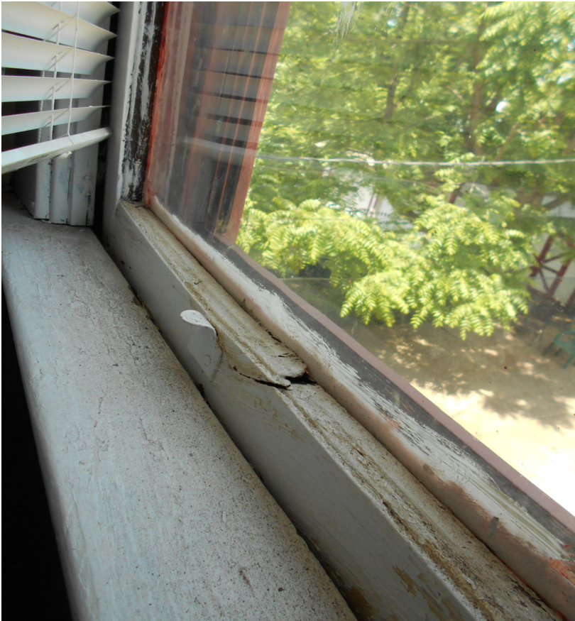
Photo 76 - Broken wooden window frame
