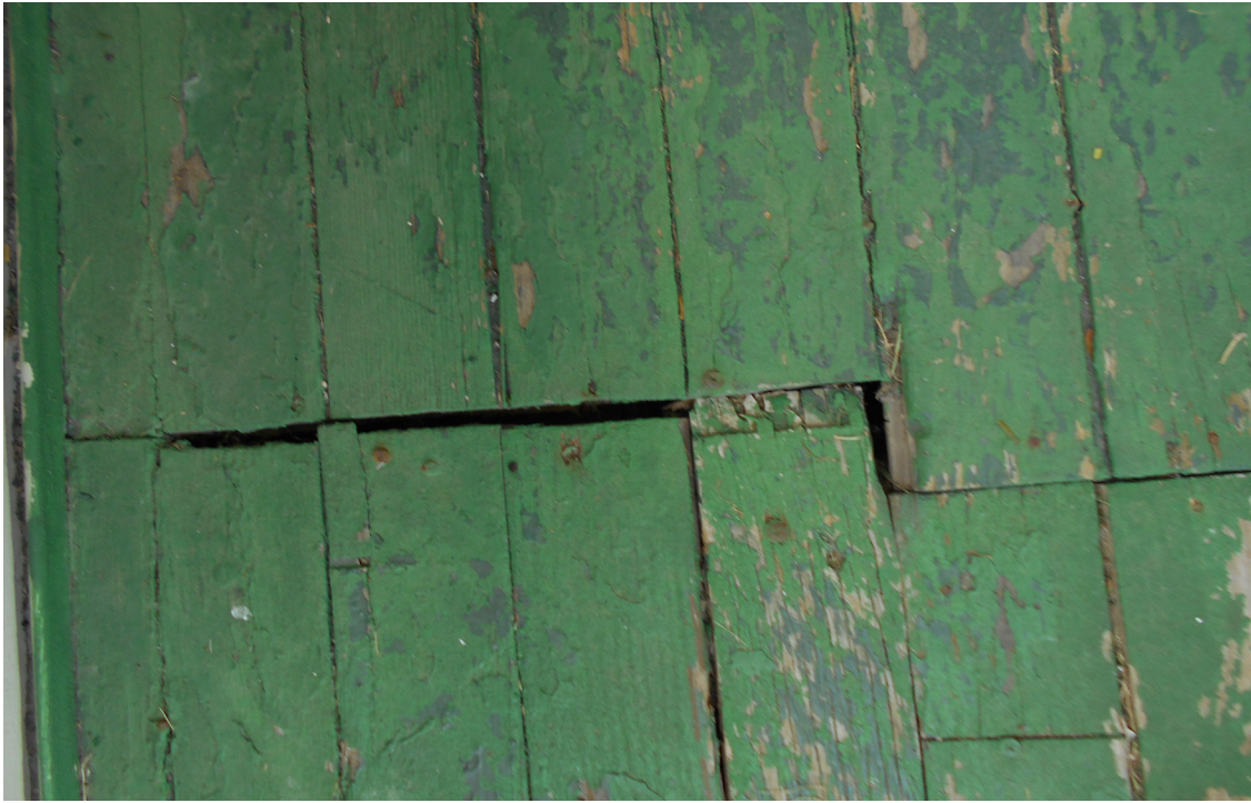
Photo 54 - Another section of the broken front porch on one of the properties
