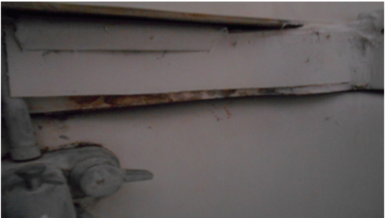
Photo 17 - Another view of the bathtub with holes/separation from bathtub and unknown black/brown substance
