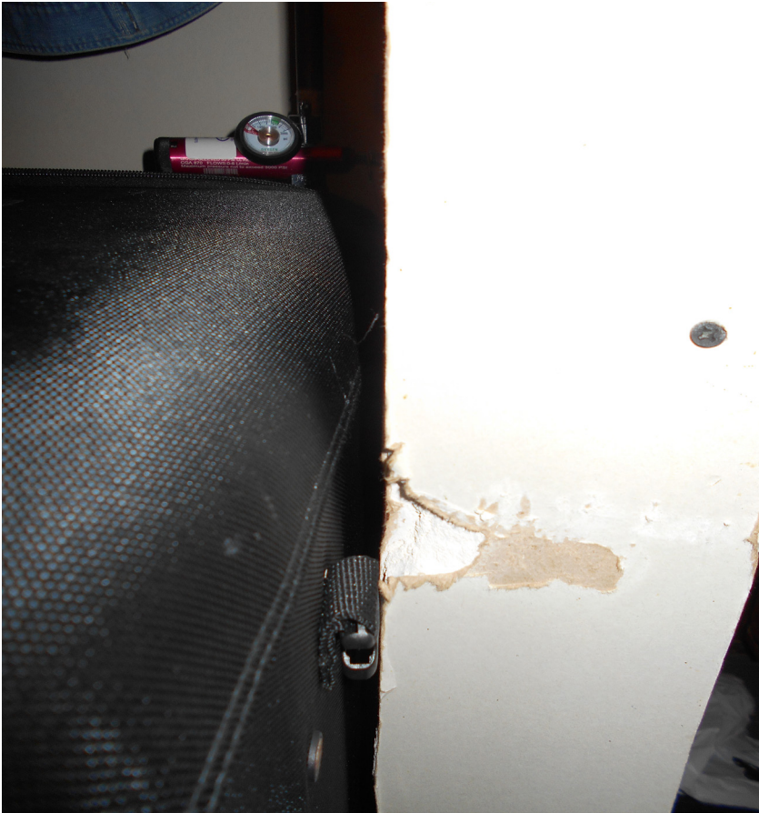
Photo 50 - A wall with a chunk of plaster missing
