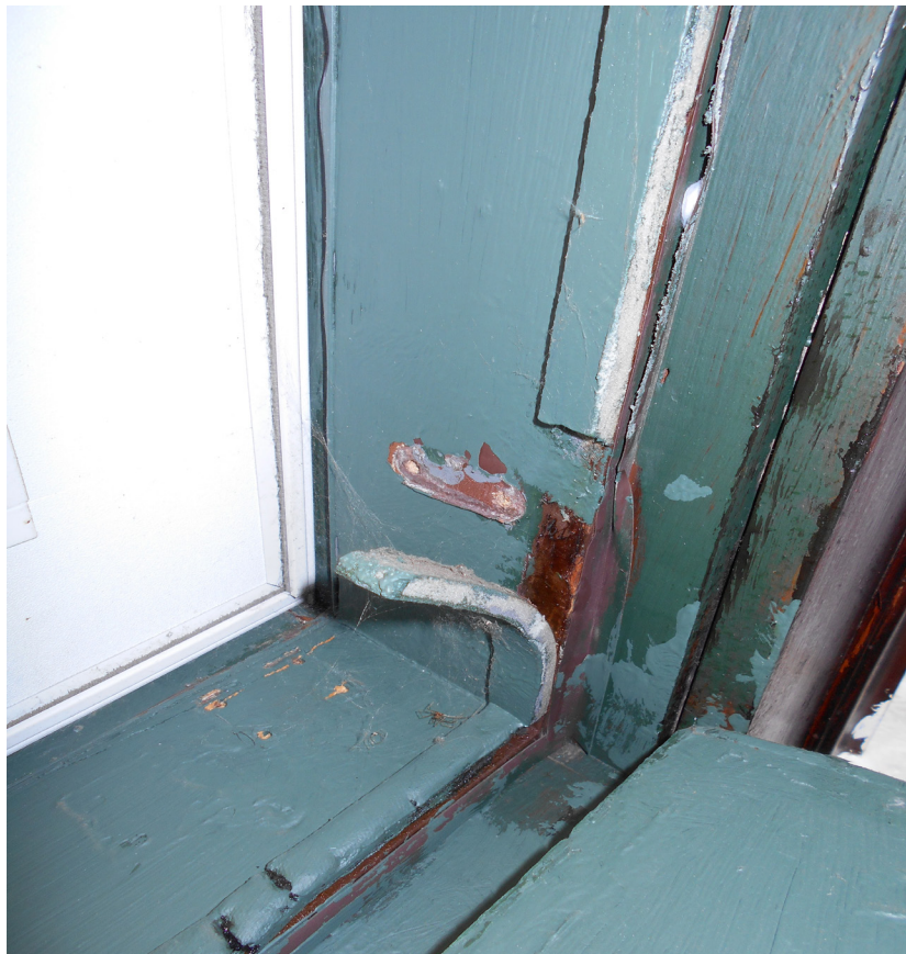
Photo 29 - Window frame peeling away from the window
