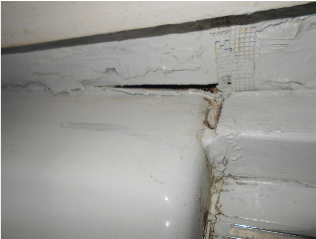
Photo 95 - Bathtub separating from wall
