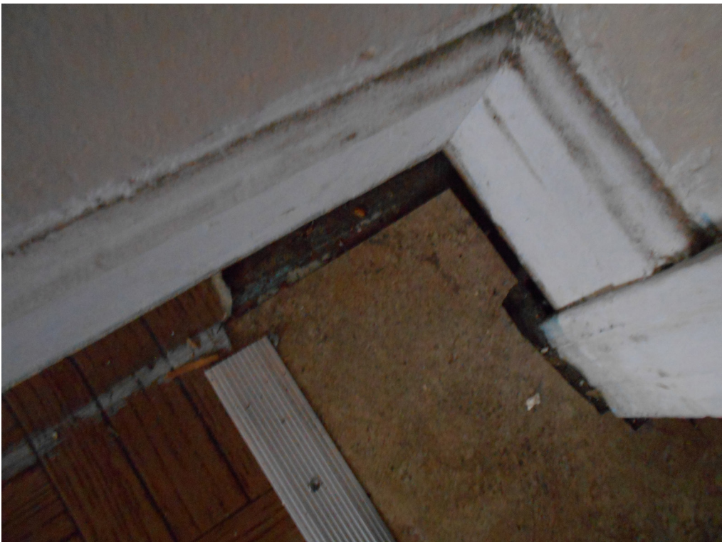
Photo 83 - Broken/missing floor
