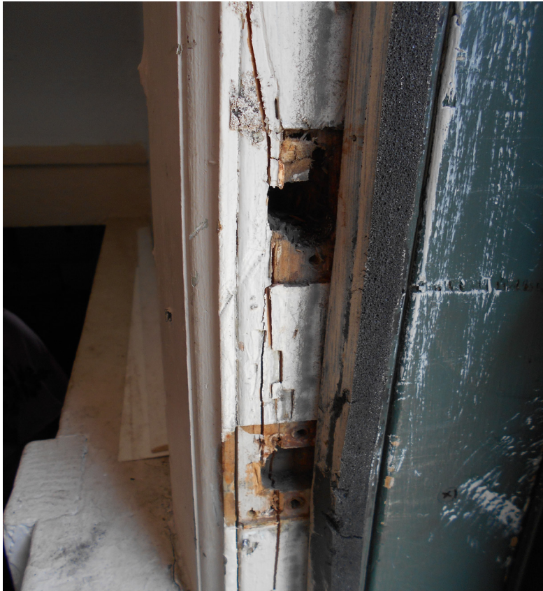
Photo 120- Door frame broken- cracking
