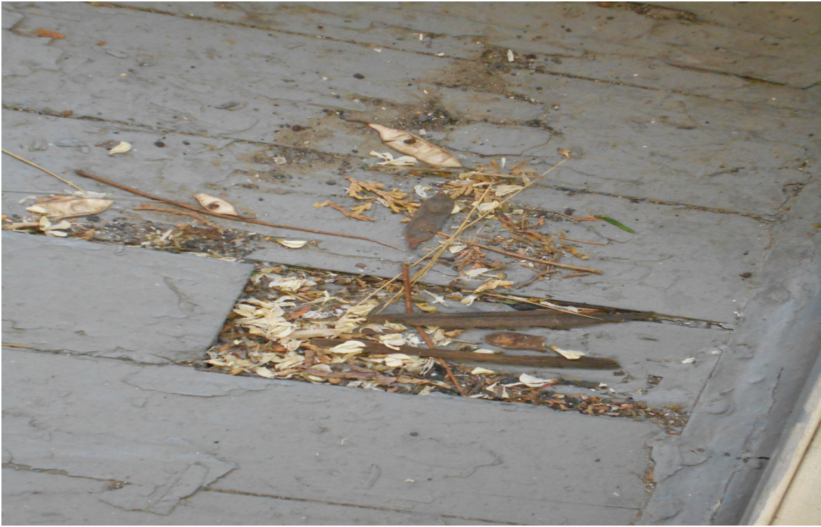
Photo 2 - Broken floorboards on porch
