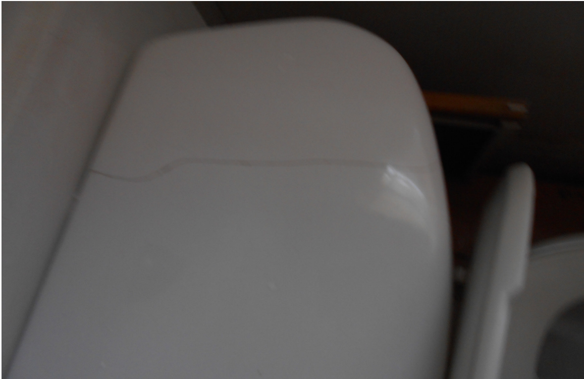
Photo 18 - Toilet is cracked
