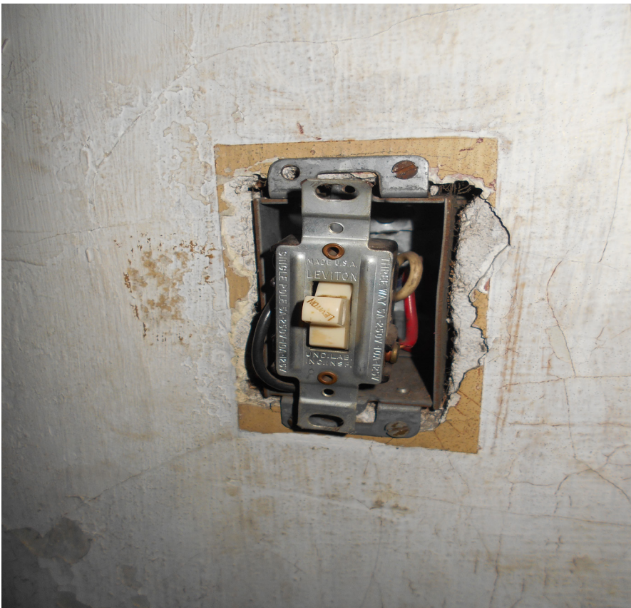
Photo 75 - Light switch without covering
