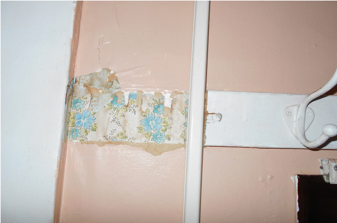
Photo20- A resident's bedroom the wall is missing paint/wallpaper/and evidence of cracks
