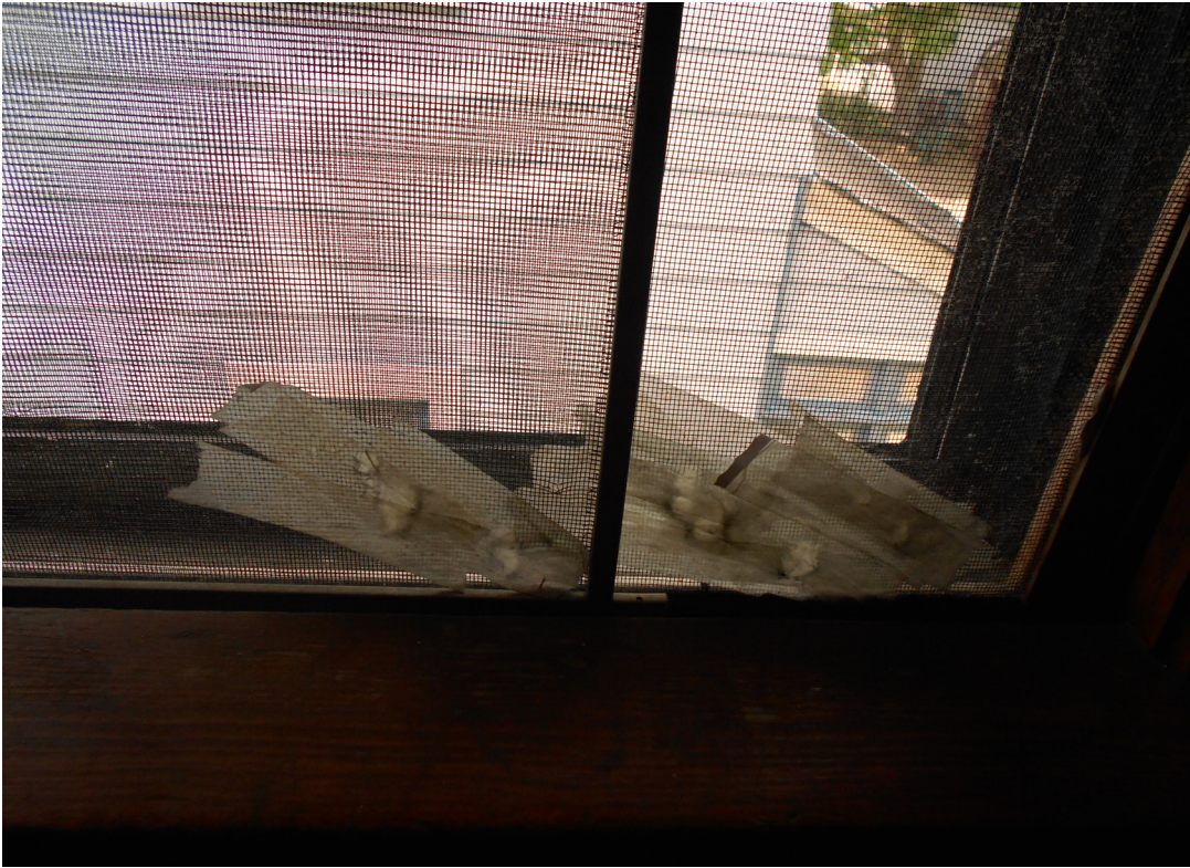
Photo 30 - Screen in a bathroom that is ripped and held together by tape
