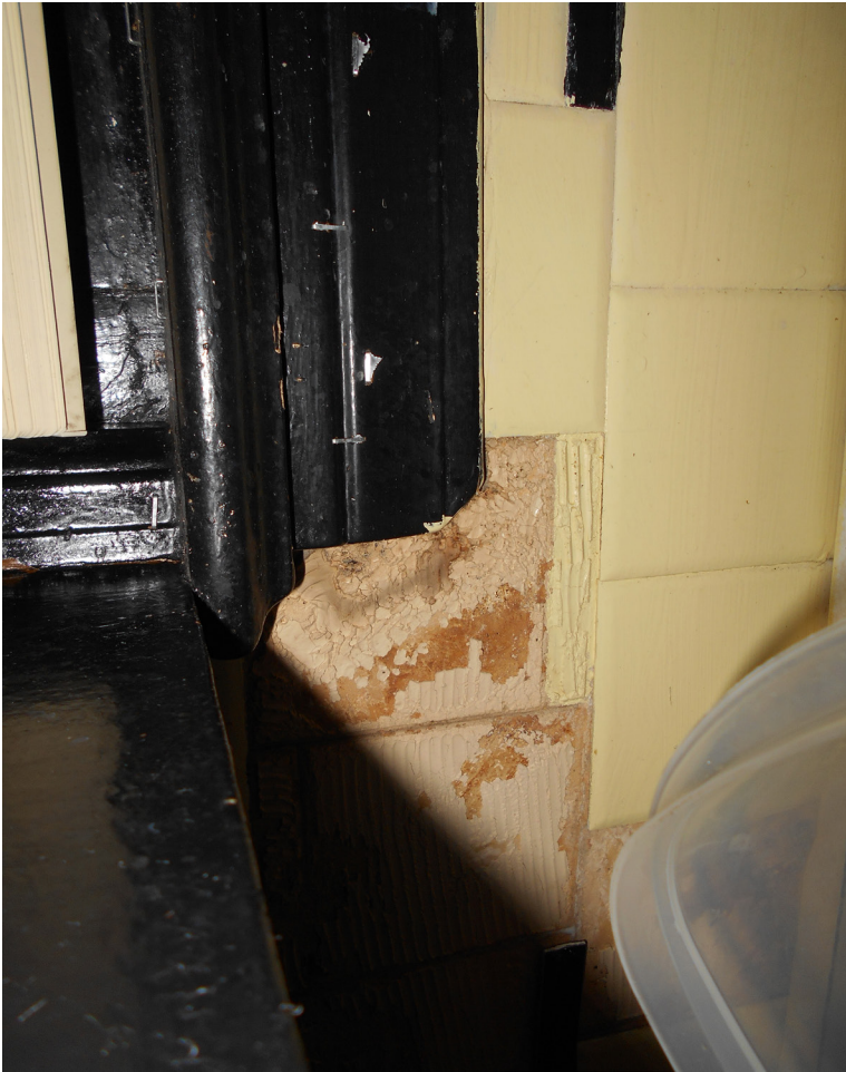
Photo 114- Missing tile in kitchen and window frame held together with staples
