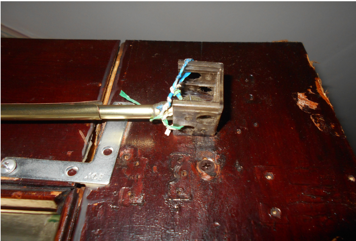
Photo 7 - Front door of one house held together by twist ties and screwed together- big crack down the middle and evidence of glue
