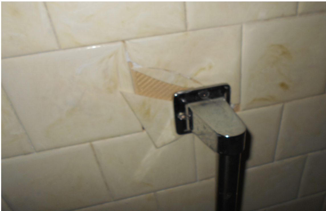
Photo 35 - Grab bar is attached to cracked tile
