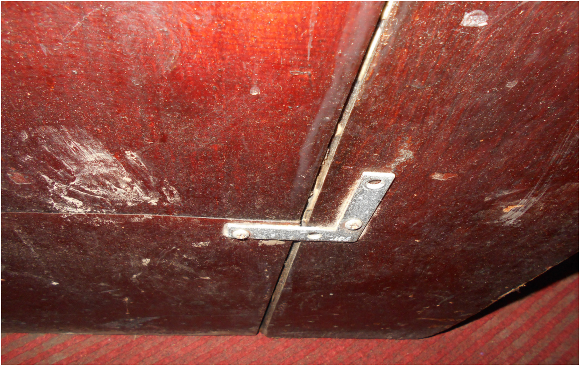
Photo 8 - Front door (bottom of door-screwed together)
