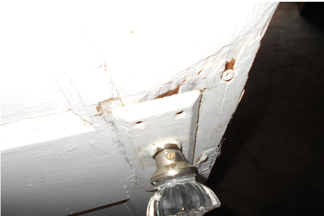
Photo 67 - Broken door with evidence of tape on the frame
