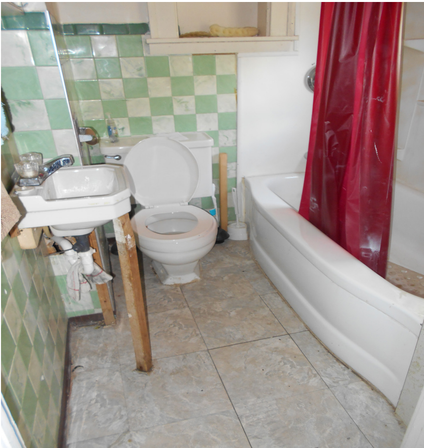
Photo 73 - A view of the resident's bathroom-sink held up by wood, hole in wall, shower curtain dirty with white substance
