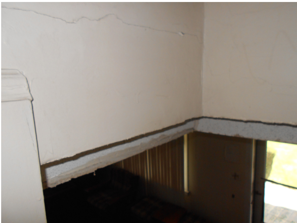
Photo 109 - Long crack in wall on stairway
