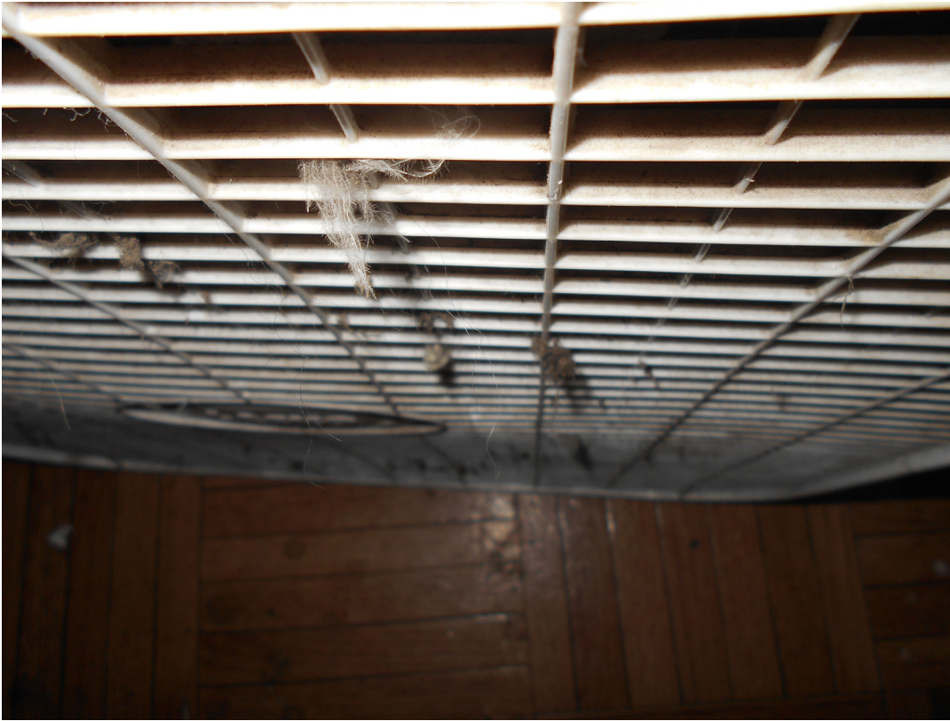
Photo 92 - Particles and caked dust in fan
