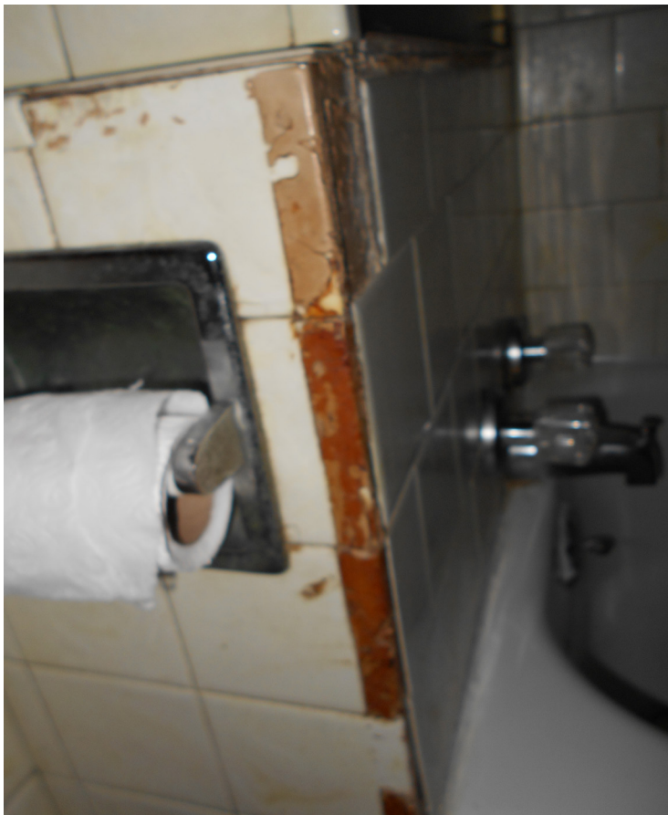
Photo 33 - Bathroom tile is missing pieces/discolored/broken
