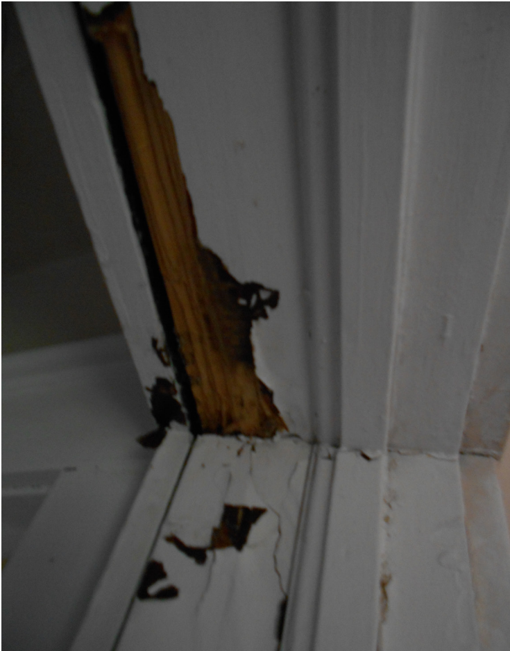
Photo 74 - Bathroom door frame that is missing pieces of wood and cracked
