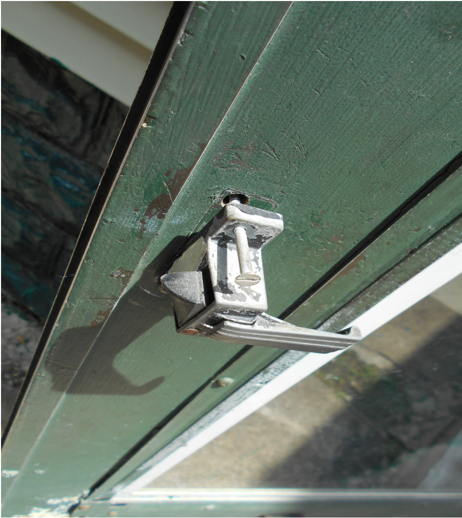
Photo 122 - Latch is detached from the door
