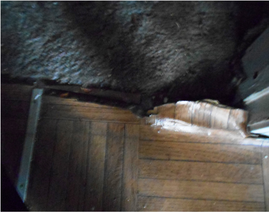
Photo 86 - Flooring that is peeling away with shards of woods exposed
