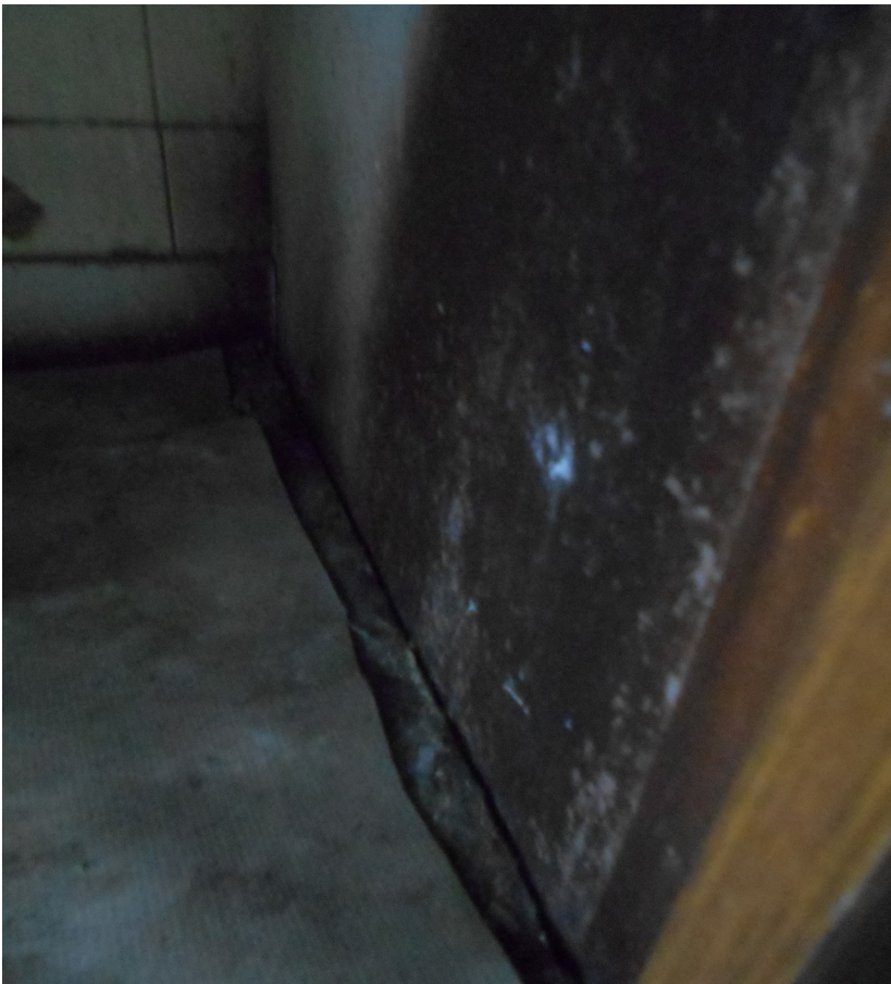
Photo 93- Bathroom floor that is peeling away
