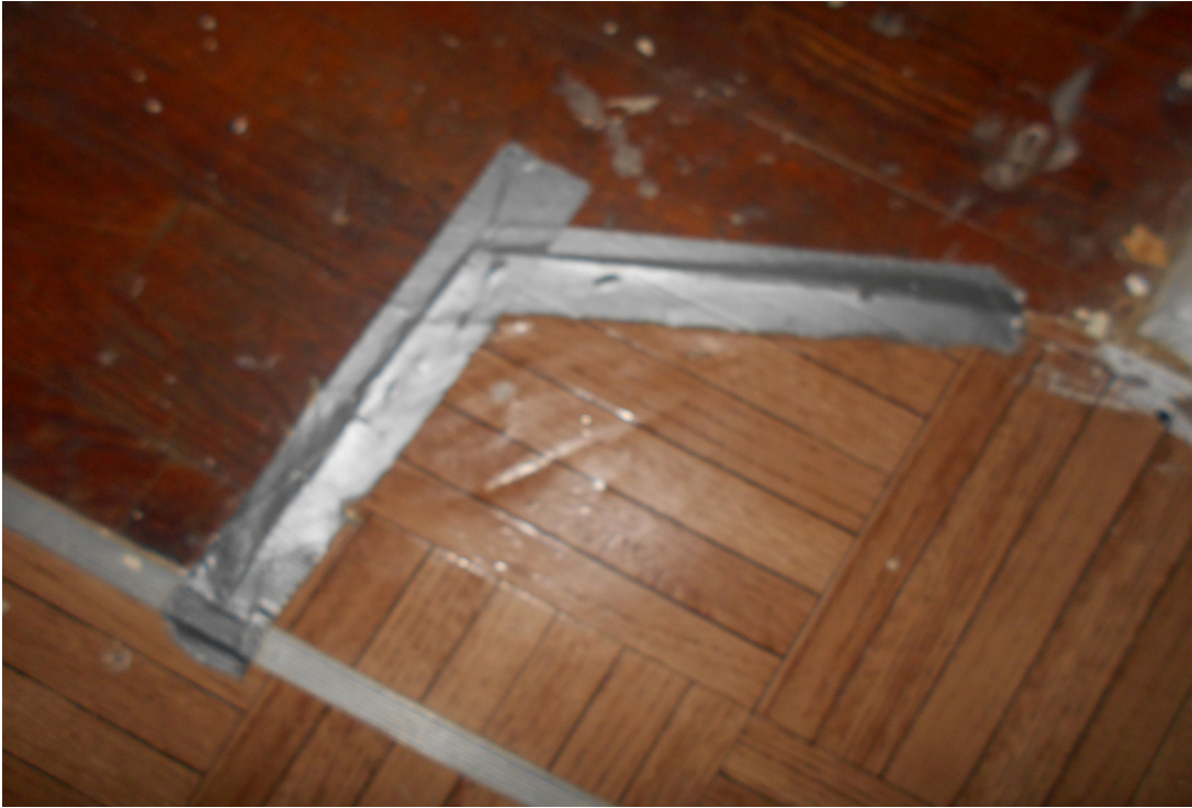
Photo 84- Floor held together by tape
