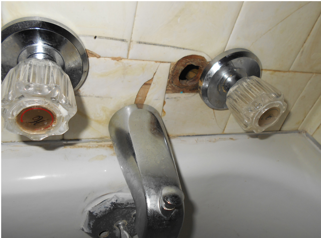
Photo 34 - Bathtub in one of the houses that has an exposed hole/cracked tile/and dirty
