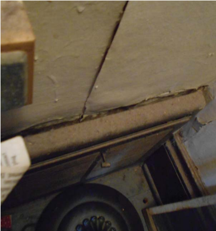
Photo 50 - Dirty-unknown particles-vent separating from wall
