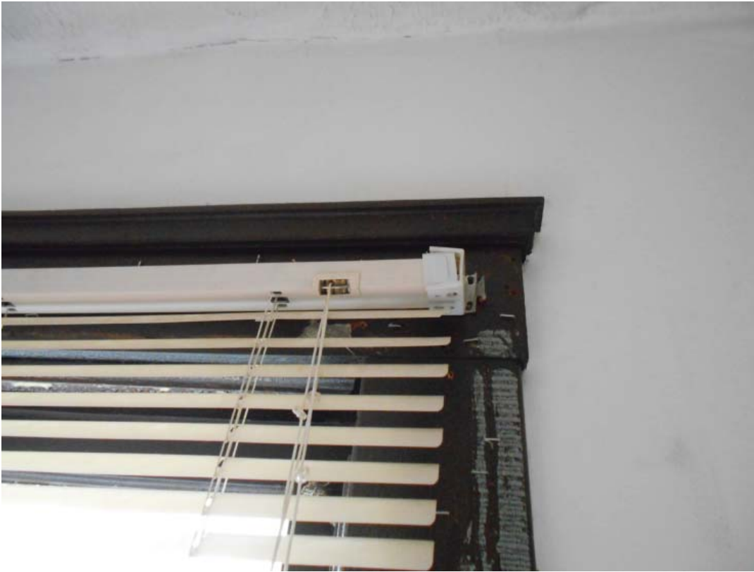
Photo 92 - Window frame covered with staples
