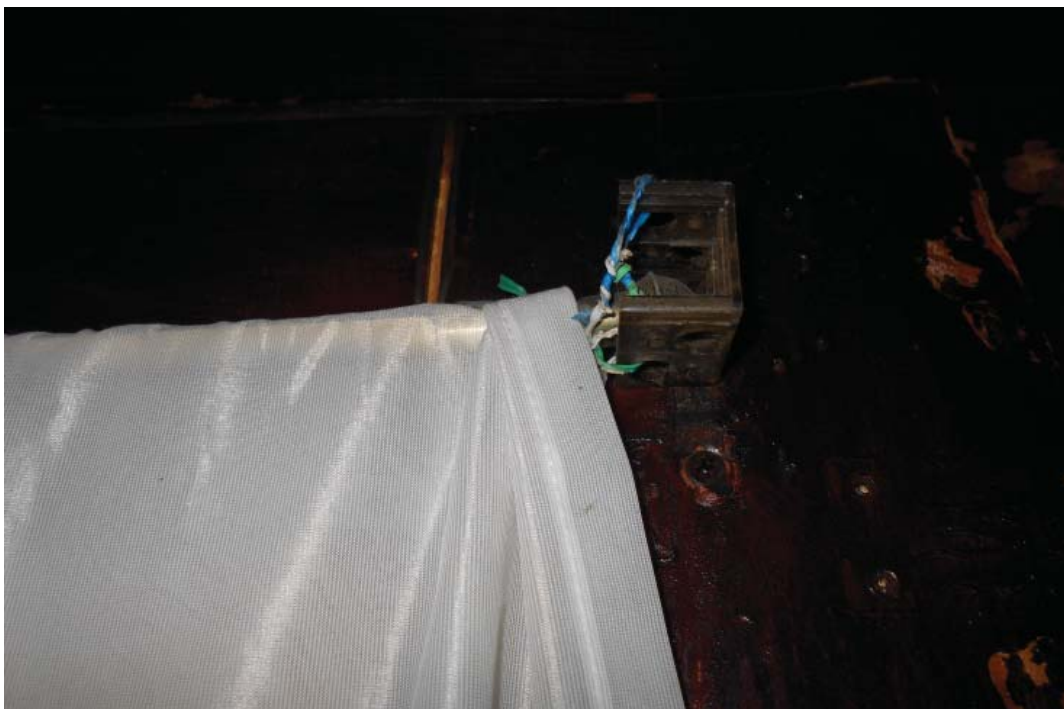
Photo 6 - Curtain hung with zip-tie, curtain holder is broken
