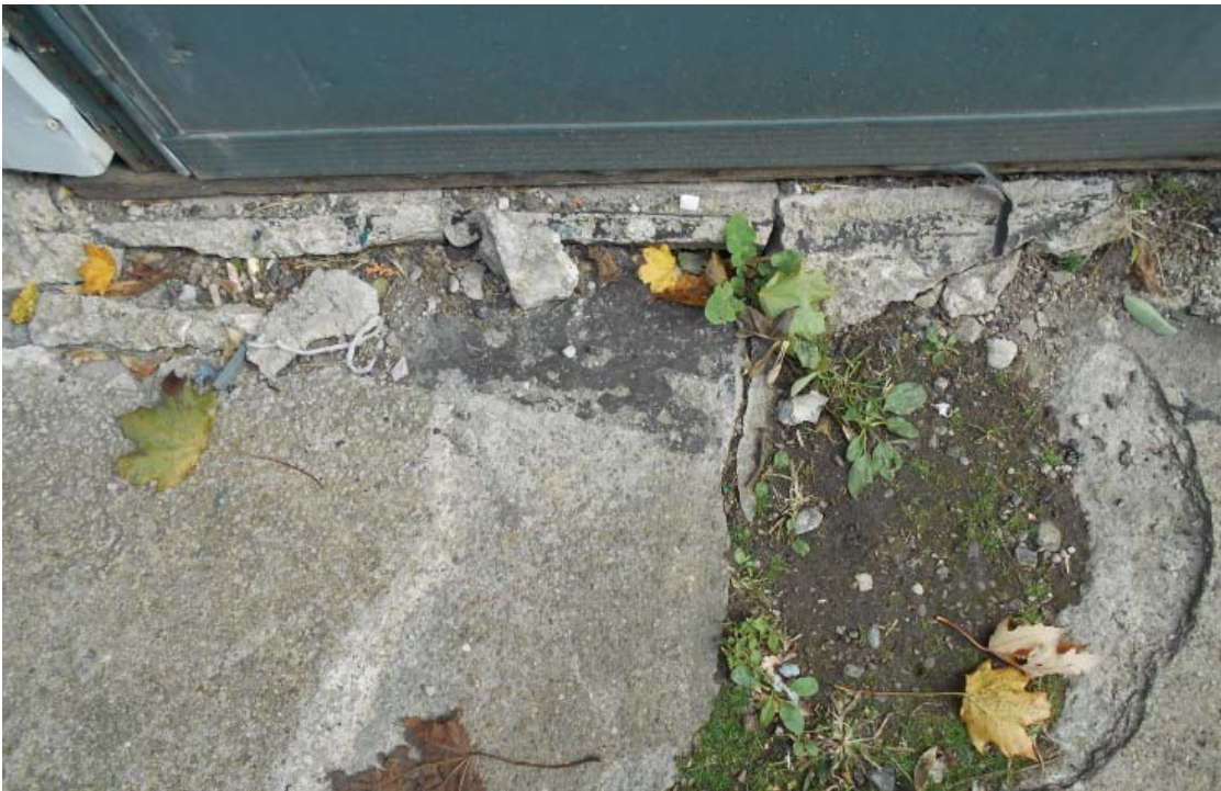
Photo 79 - Broken cement outside door-safety issue
