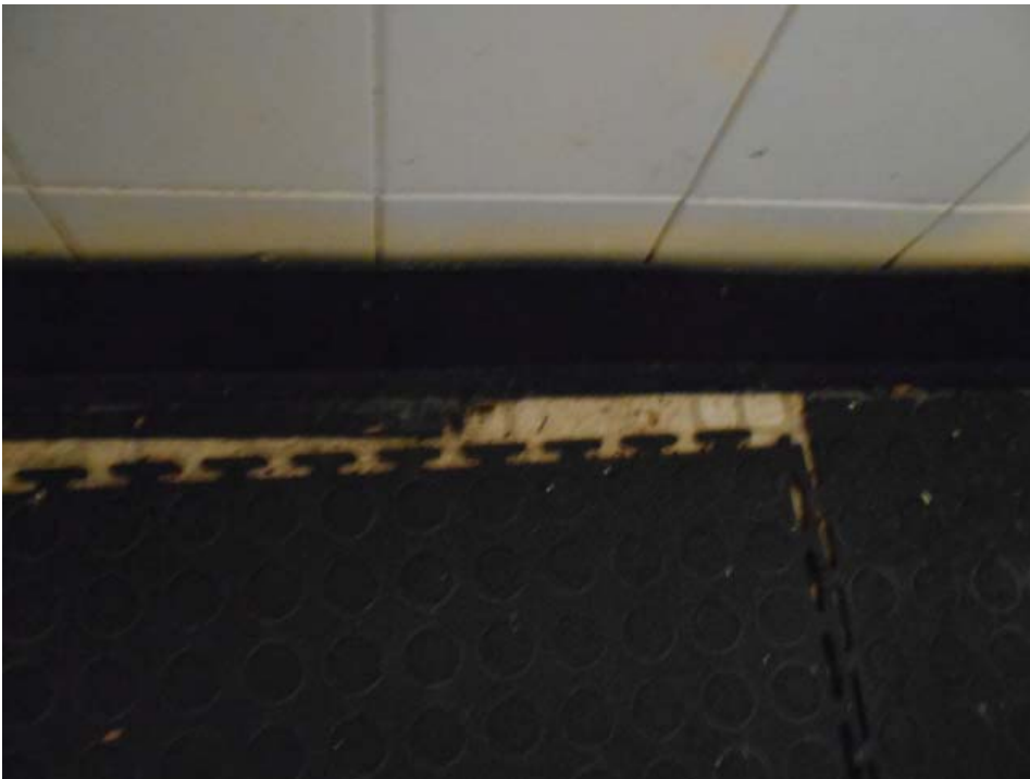
Photo 63 - Bathroom flooring-ripped-torn
