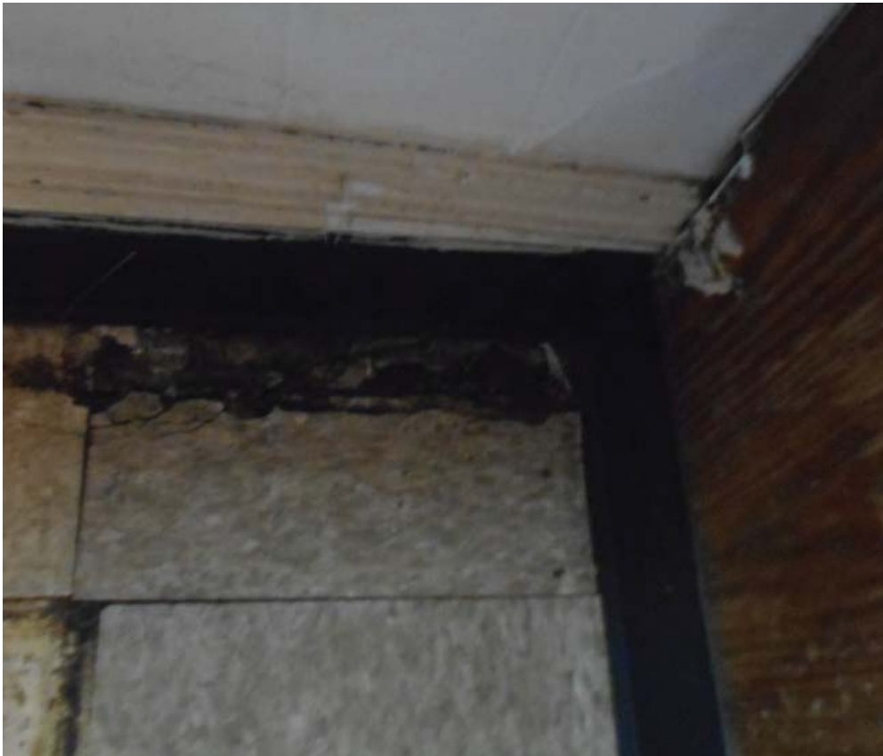
Photo 10 - Broken/ missing tile-dirty/ unknown black matter
