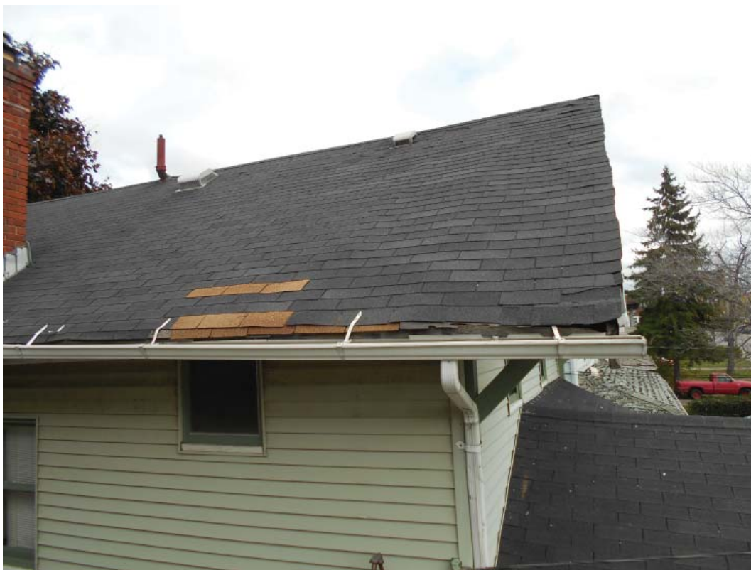
Photo 32 - Shingles lifting up from roof
