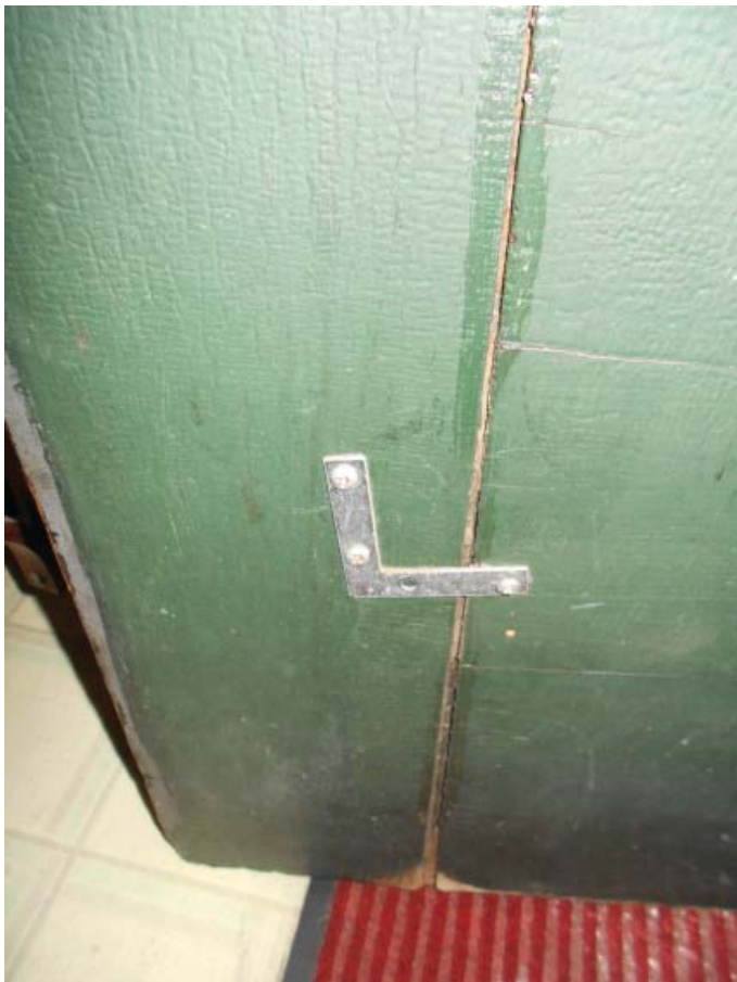
Photo 4 - Front door broken-held together with clamp
