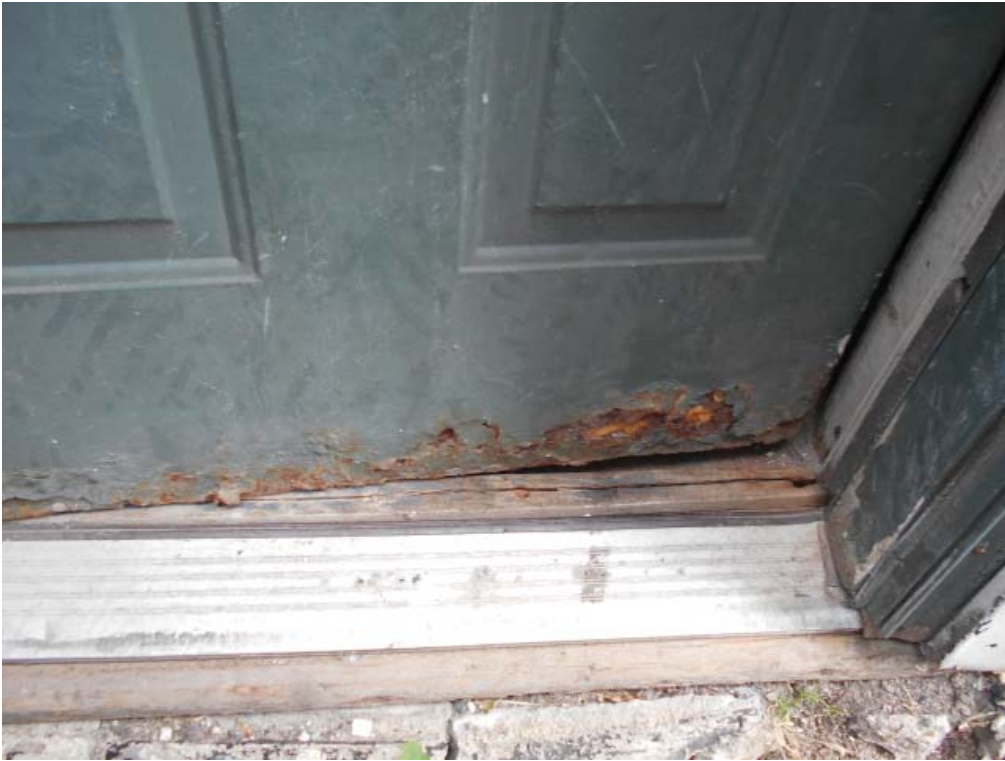
Photo 76 - Rusted door with hole
