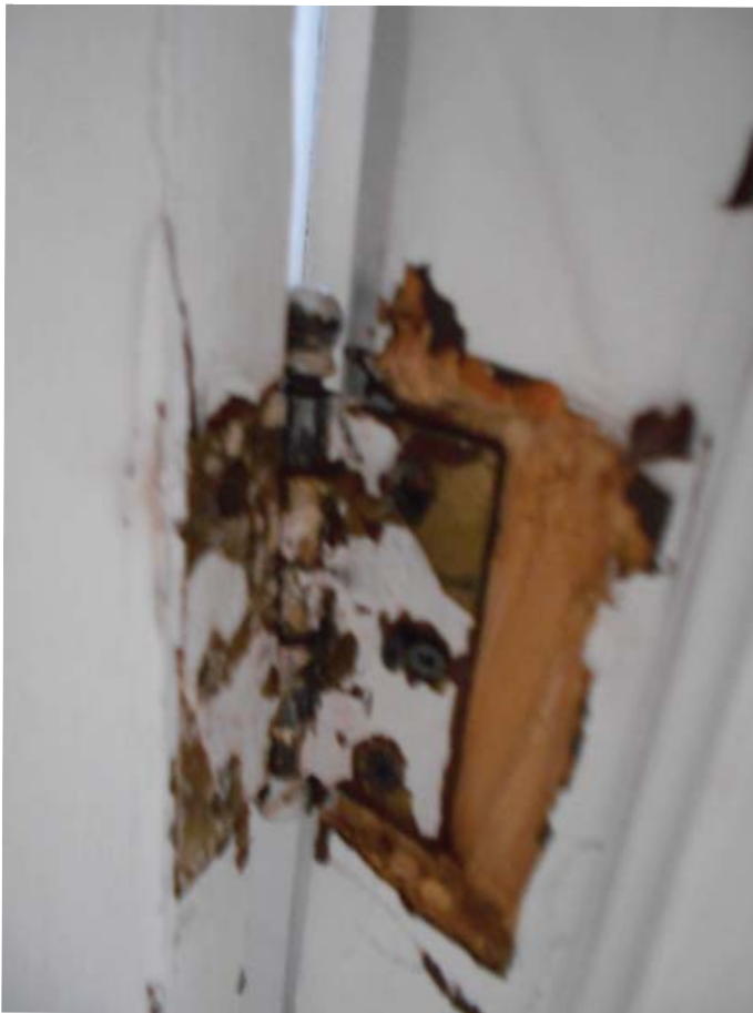
Photo 84- Door hinge-broken- rusted
