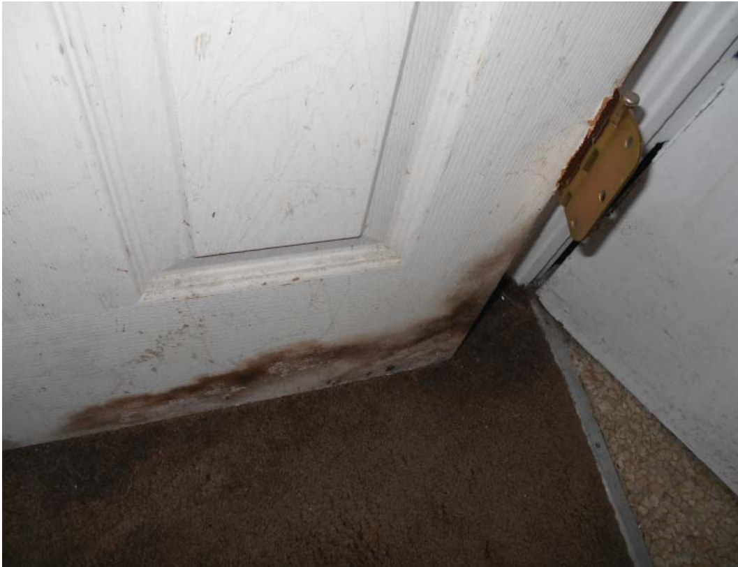
Photo 98 - Broken door with stained/black matter
