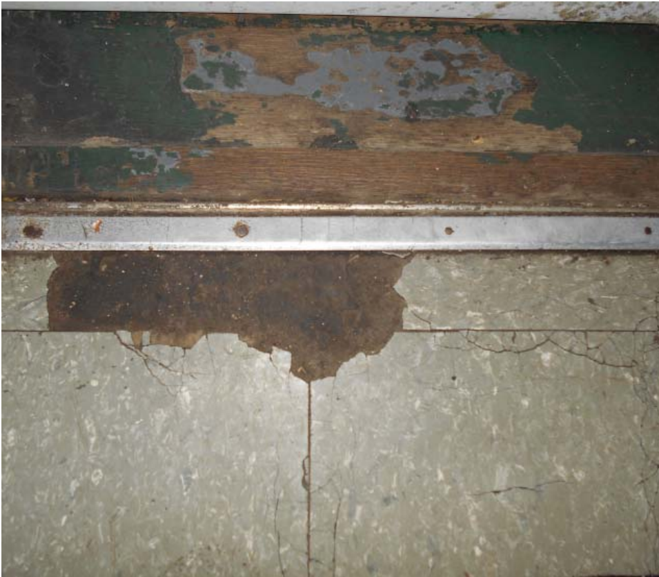
Photo 12 - Floor tile missing-wood missing-cracked- dirty
