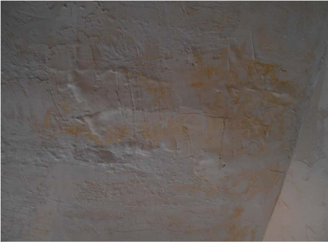
Photo 102- Staining on ceiling with cracks
