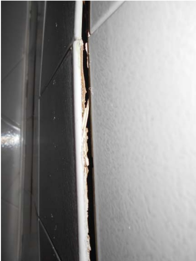
Photo 66 - Bathroom tile pulling off of the wall
