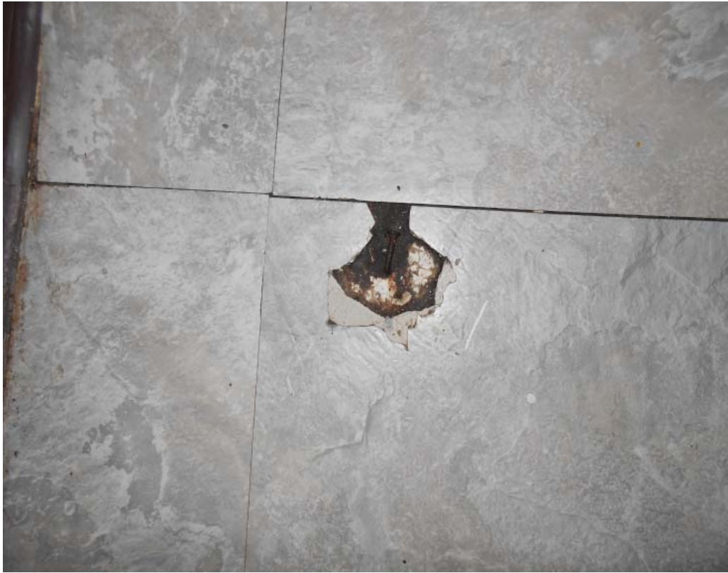
Photo 88 - Broken tile with hardware in the bottom
