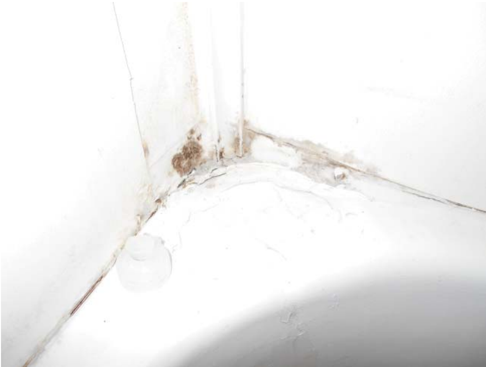
Photo 68 - Bathtub with unidentified black matter-cracked
