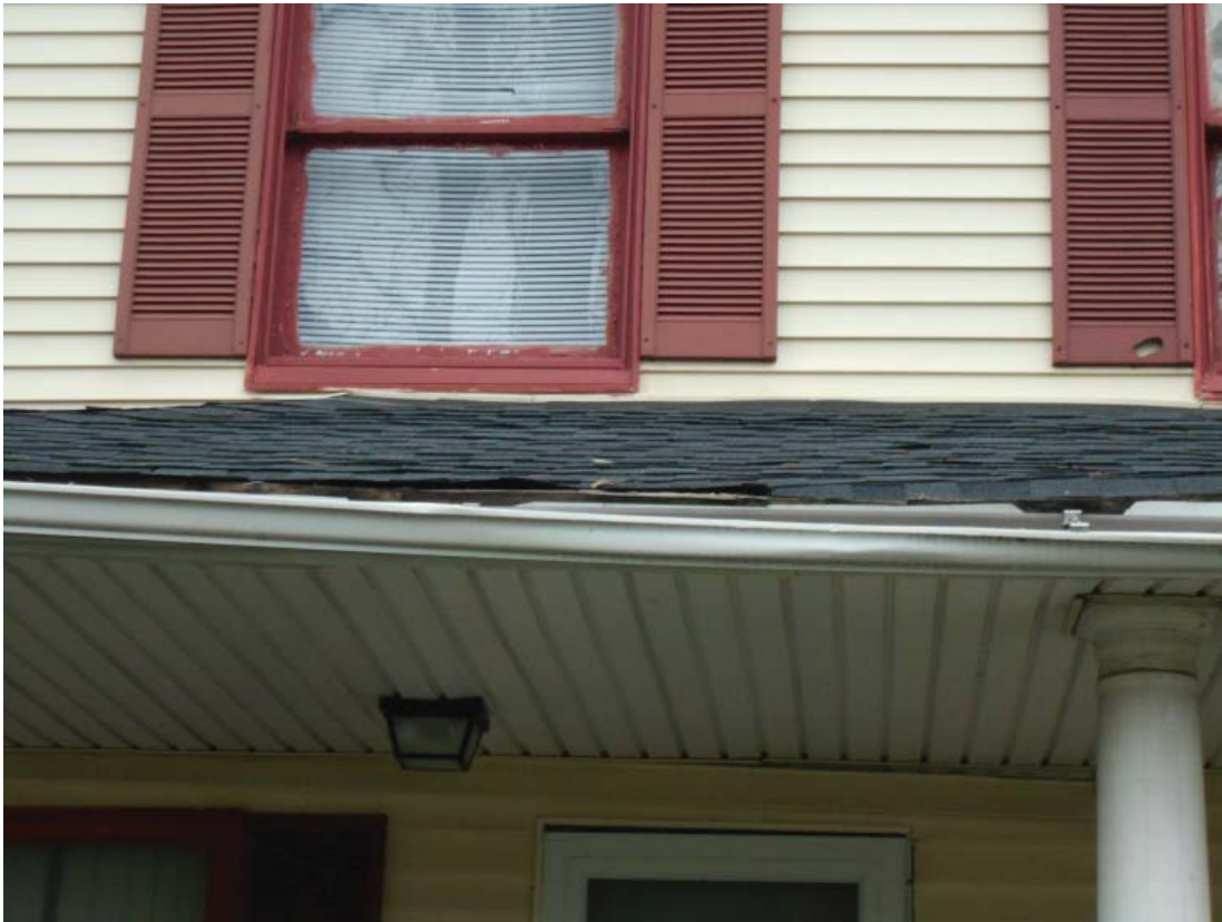
Photo 1 - Gutter separating from roof, roof shingles loose
