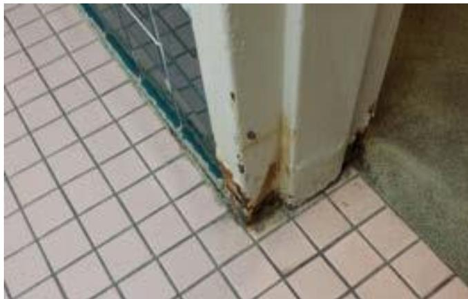
Holes in door frame, rust in door frame, black mold in flooring tiles
