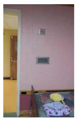
Inaccessible Light Switch at Approx 5 feet six inches
