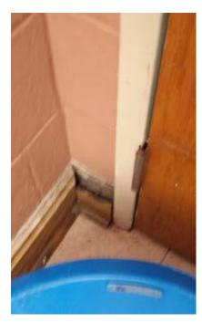
Missing Floor Board and Black Mold
