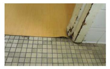
Damaged Rusty Doorway, Black Mold on Floor, Warped Flooring
