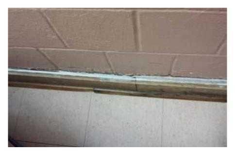
Damaged Floor Board and Black Mold
