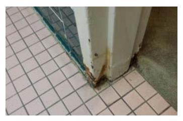
Holes in door frame, rust in door frame, black mold in flooring tiles
